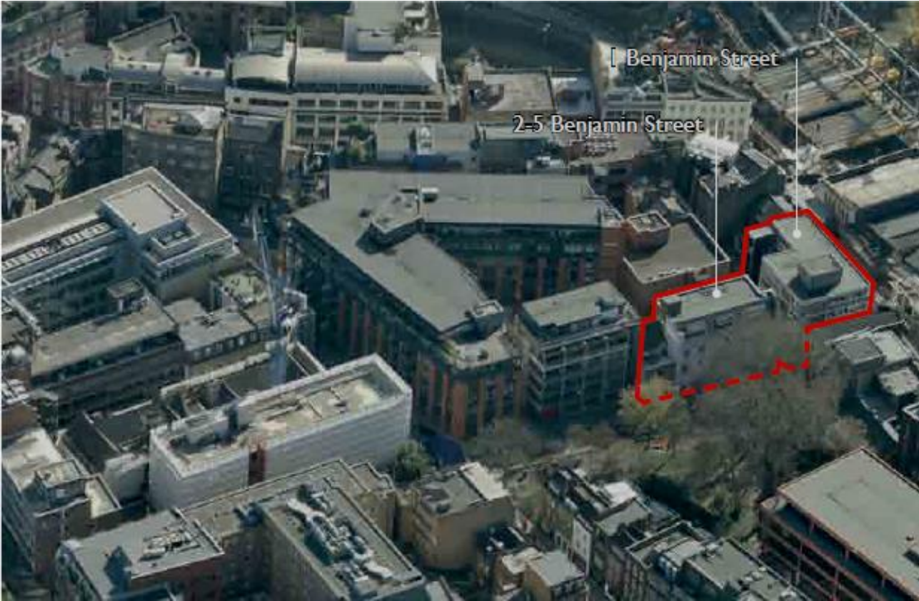
Photo 2: Aerial view from North
